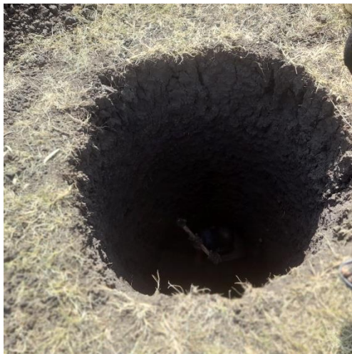
RIEKO borehole at the initial stage
