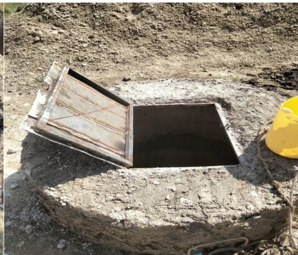
RIEKO borehole towards completion
