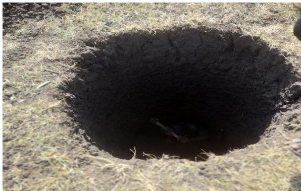
RIEKO borehole at the initial stage
