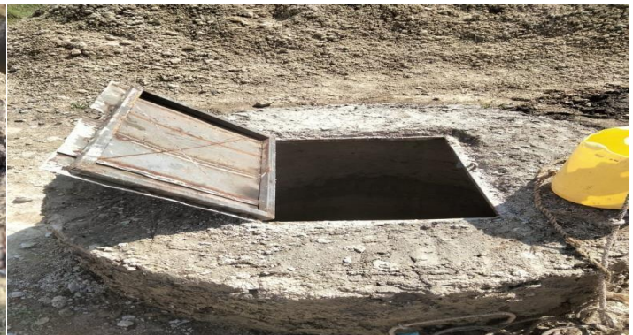
RIEKO borehole towards completion
