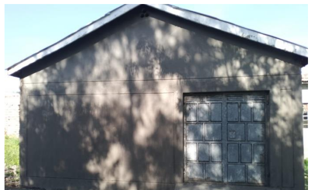
Final posho mill hall
