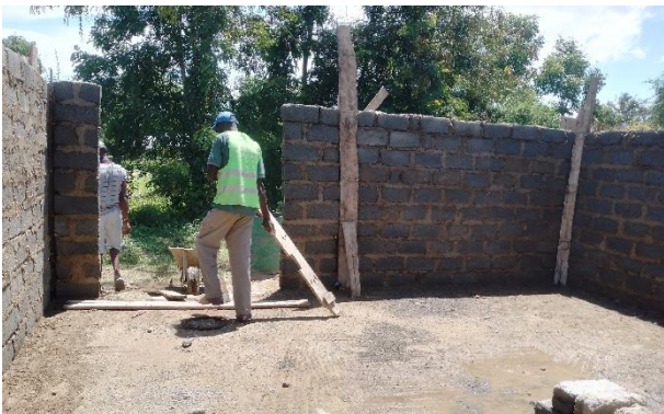
Initial construction of posho mill hall
